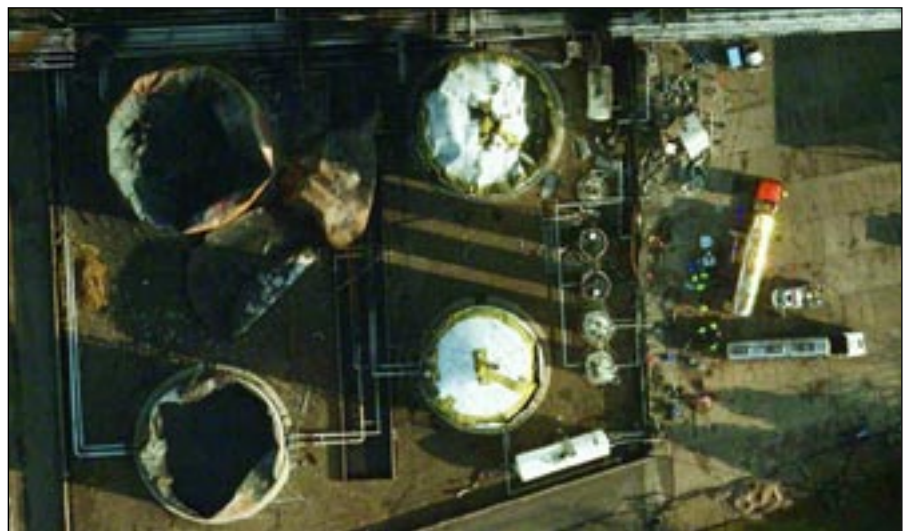
Buncefield Oil Depot, January 2006 Image from Cities Revealed™ aerial photography © The GeoInformation Group, 2006
